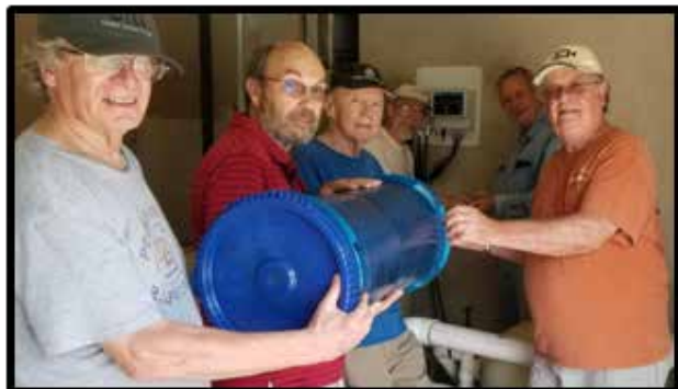
Attaching cover plate at pool building
