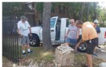
Cleaning up the column debris at Barker Cypress & Oakhampton
